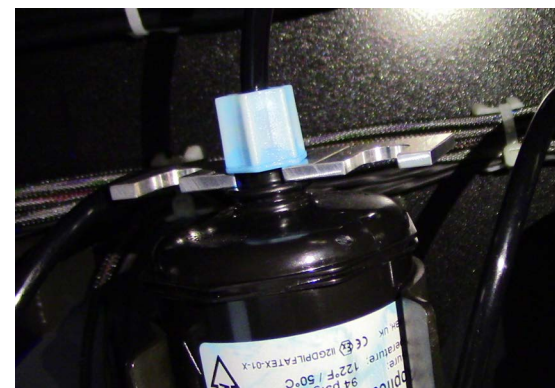
Figure 11-5 Proper positioning of gauge on filter
